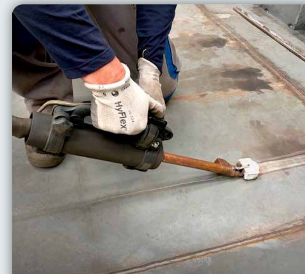
SHIPYARD - HEAT SHRINKING - CONSTRUCTION NAVALE - CHAUDRE DE RETRAIT Large L20/B4 Powerduction 220LG
